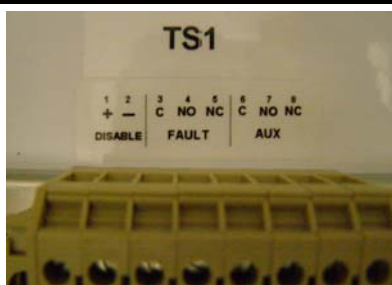
Figure 3-4: Typical Control Connections at TS1
