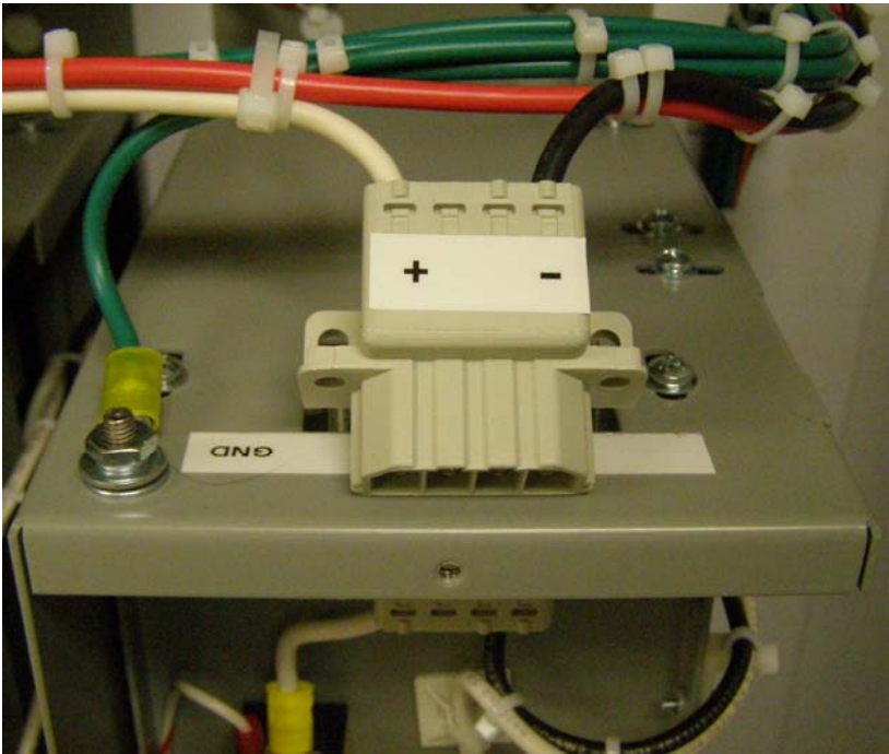
Figure 5-2: Battery Module Plug Connected
