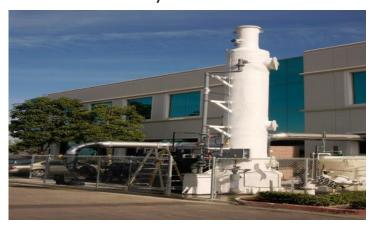
Ross Incineration Systems manages both hazardous and non-hazardous wastes. The design of the waste handling equipment and the incinerator itself allows for maximum flexibility in the types of wastes and containers that can be managed for incineration. The incineration system uses both a rotary kiln and a custom designed main chamber system to assure flexibility in handling even the most difficult to manage wastes.
